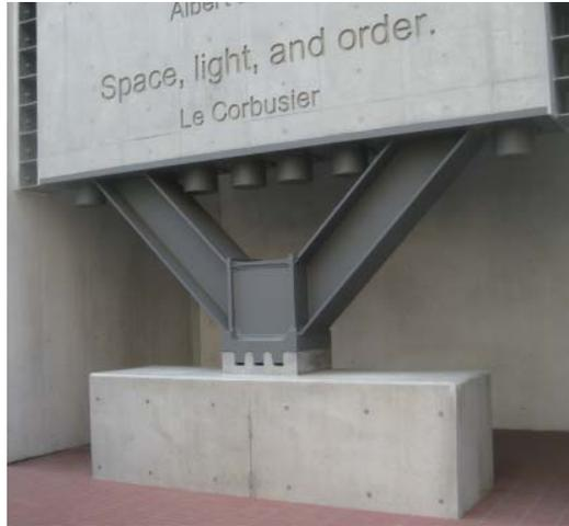
Figure 2. Cast iron base hinge to prevent shock damage
